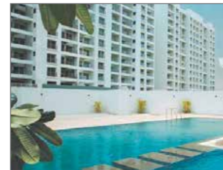
GODREJ HORIZON NIBM ANNEX, PUNE Completed in 2015
